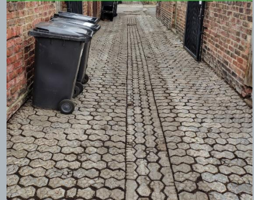
After ✓ vegetation removed Area tidied up
