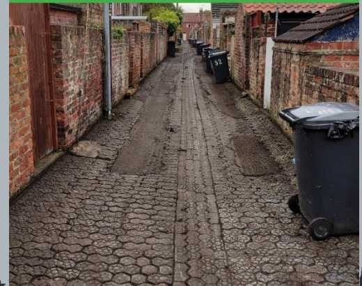
After ✓ vegetation removed Area tidied up
